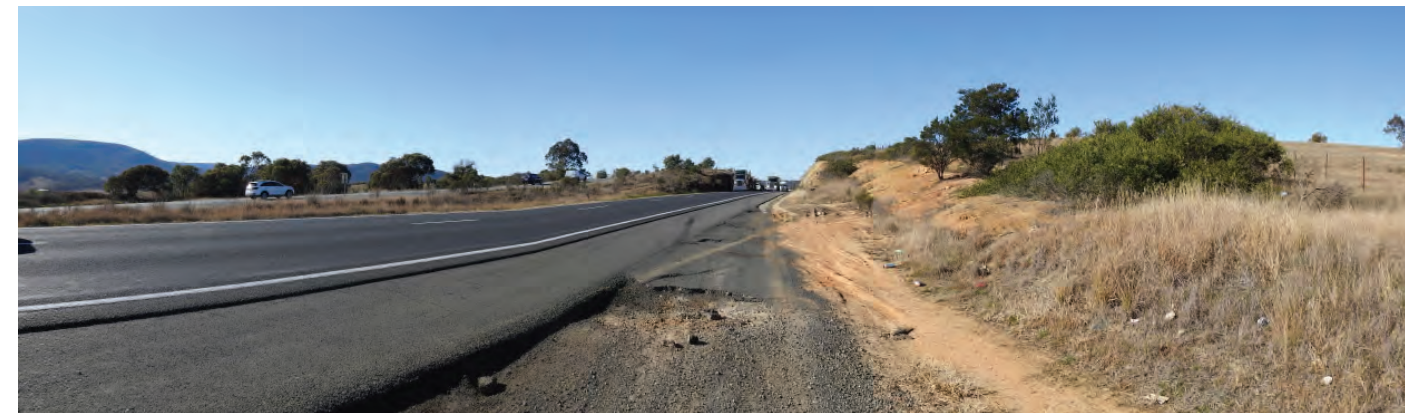
Image 4 Hume Highway looking east
