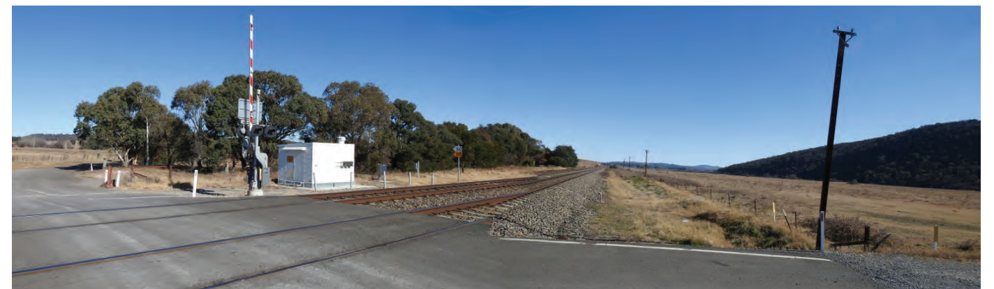
Image 12 Rail corridor (Main Southern Railway Line) looking east from Murrays Flat Road crossing
