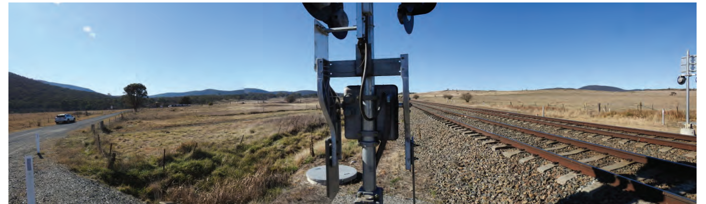
Image 11 Rail corridor (Main Southern Railway Line) looking east from Murrays Flat Road crossing
